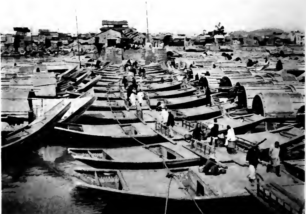
The central portion of the famous bridge of Chauchowfu is made up of boats that swing aside when passage up or down the river is needed
